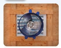
**Wide Mount:** The AFG can be mounted on a wide louver, but additional mounting steps must be taken in order for the fan to work properly. As shown in Figure 2.1B, two additional boards must be fastened to the boards framing the gable vent so the AFG can be mounted securely. Use 3 All-Purpose screws per tab.
